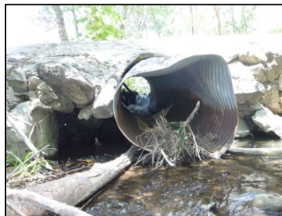
Figures 24 – 26. Osborn Road Crossing with damaged and debris filled culverts
