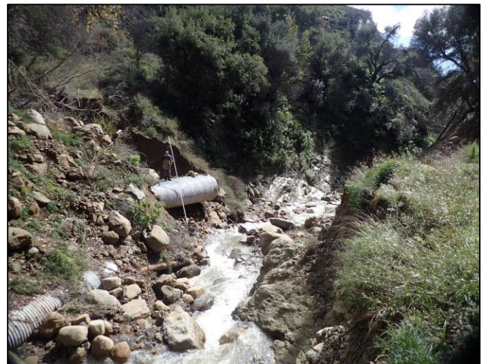
Figure 68. Upstream view of blow out forest service road on West Fork El Capitan Creek.
