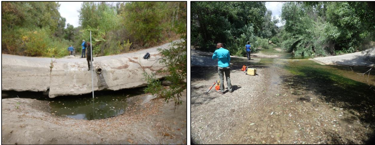
Figures 31 & 32. Fraser Street low-water crossing prior to (left) and after sedimentation (right).
