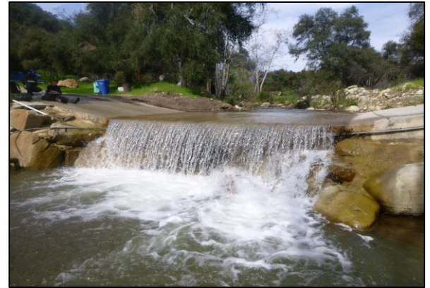
Figure 23. Private road low-water crossing on Sisar Creek.
