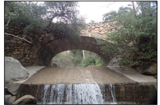
Figure 72. View of outlet apron and plunge point at Las Canoas Road crossing on Rattlesnake Creek.
