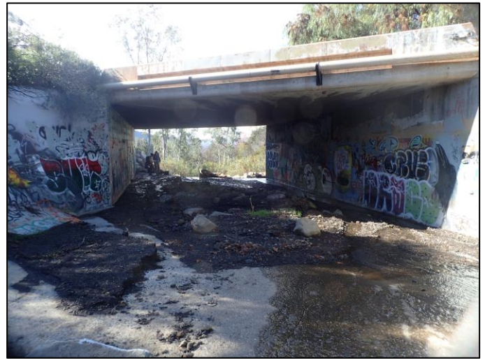
Figure 47. Upstream view of concrete lined inlet apron at the McAndrew Road crossing.
