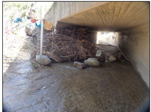
Figure 61. Debris at inlet of CAN_002_R Hwy 33 crossing.
