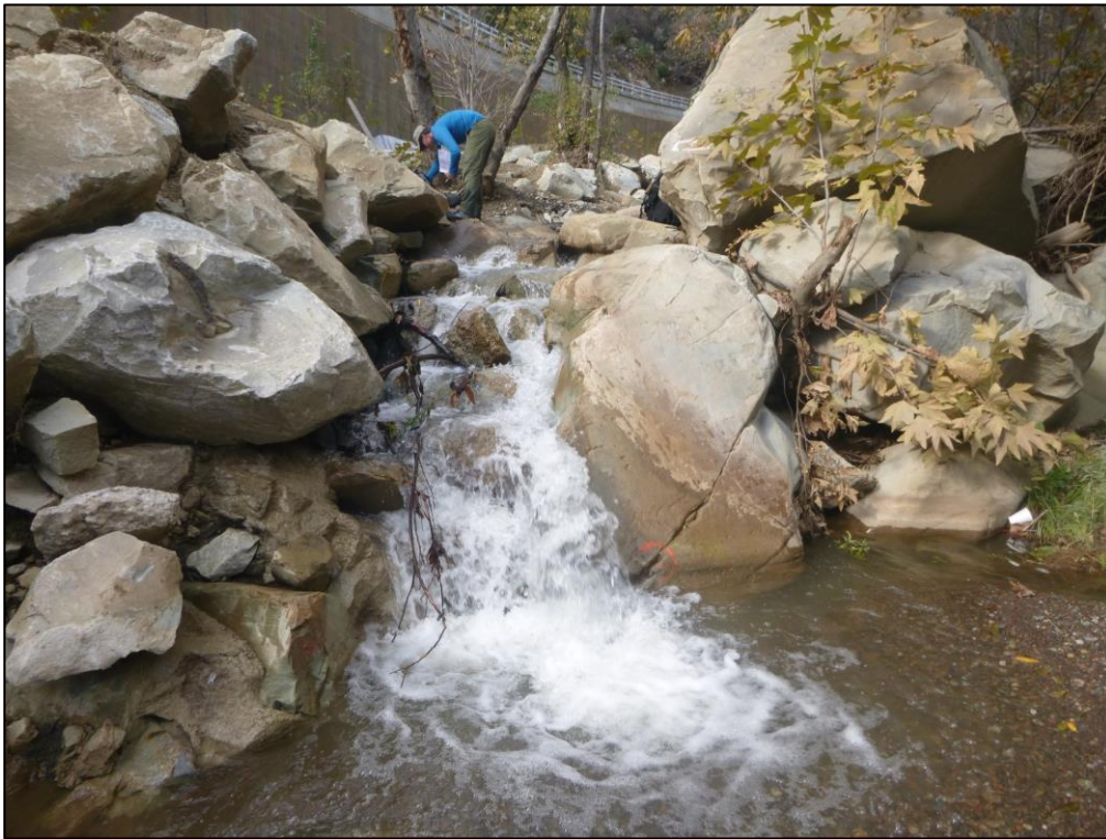
Figure 51. Downstream view of boulder riprap grade control on North Fork Matilija Creek.
