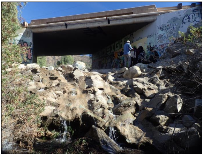
Figure 46. Downstream view of concrete boulder riprap outlet apron at the McAndrew Road crossing.
