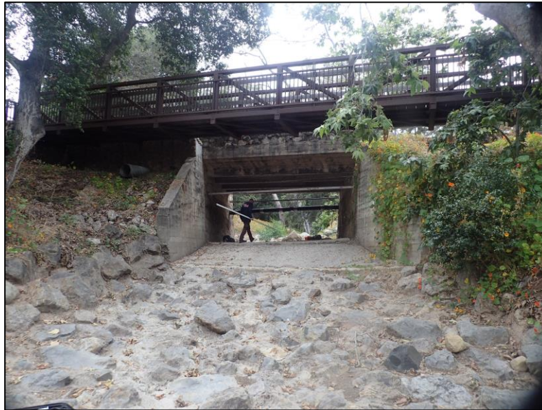
Figure 89. View of boulder and concrete outlet apron at Santa Rosa Lane crossing on Oak Creek.
