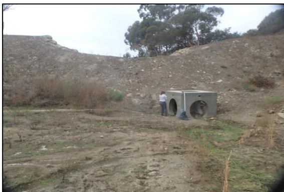
Figure 102. Drainage intake for debris basin on Romero Creek.
