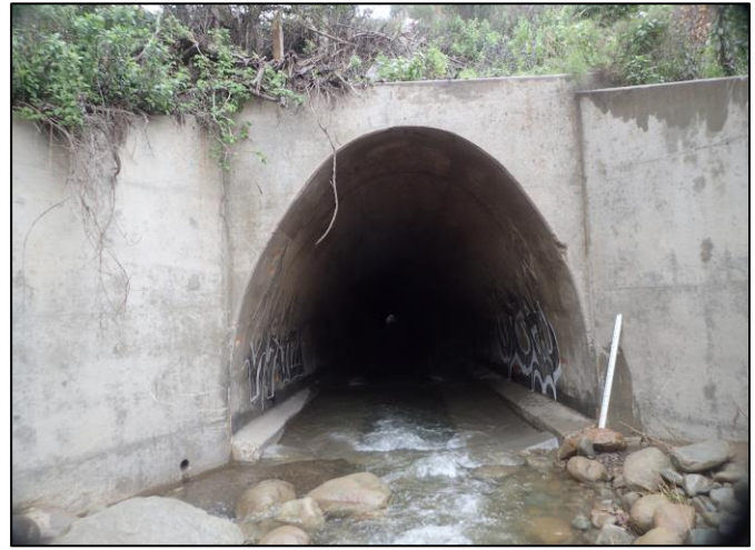
Figure 65. View of culvert inlet and weir at Hwy 101 El Capitan Creek crossing.
