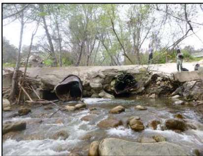
Figures 24 – 26. Osborn Road Crossing with damaged and debris filled culverts
