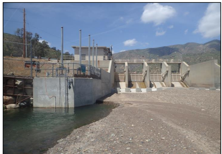
Figure 30. Downstream view of Robles Diversion Dam. Fish ladder entrance is located at the left of image, in the wetted portion of channel.
